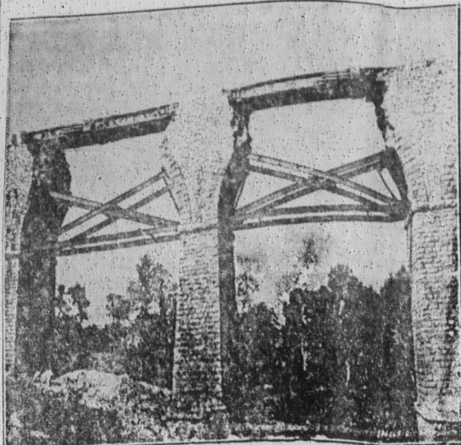
Four days later P. de l'Arc was repaired and trains were in operation carrying stores and munitions to advancing American troops.
