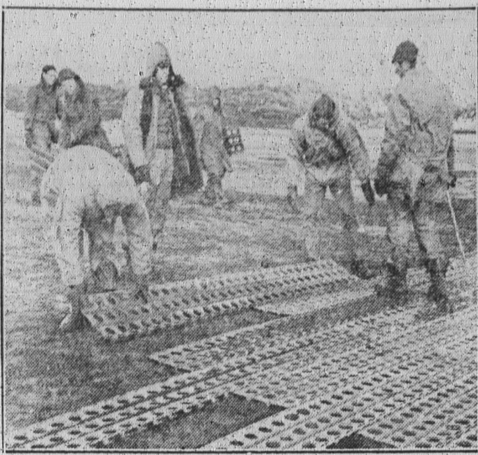
Bureau of Public Relations, U. S. War Department AVIATION ENGINEERS IN THE ARCTIC —A vital link in the chain of air bases built by U. S. Aviation Engineers is this landing field somewhere in the Aleutians. The field having been cleared, graded and rolled, portable steel landing plank is laid to complete the intricate system of runway and taxiways from which our aircraft will carry the war to the enemy.
